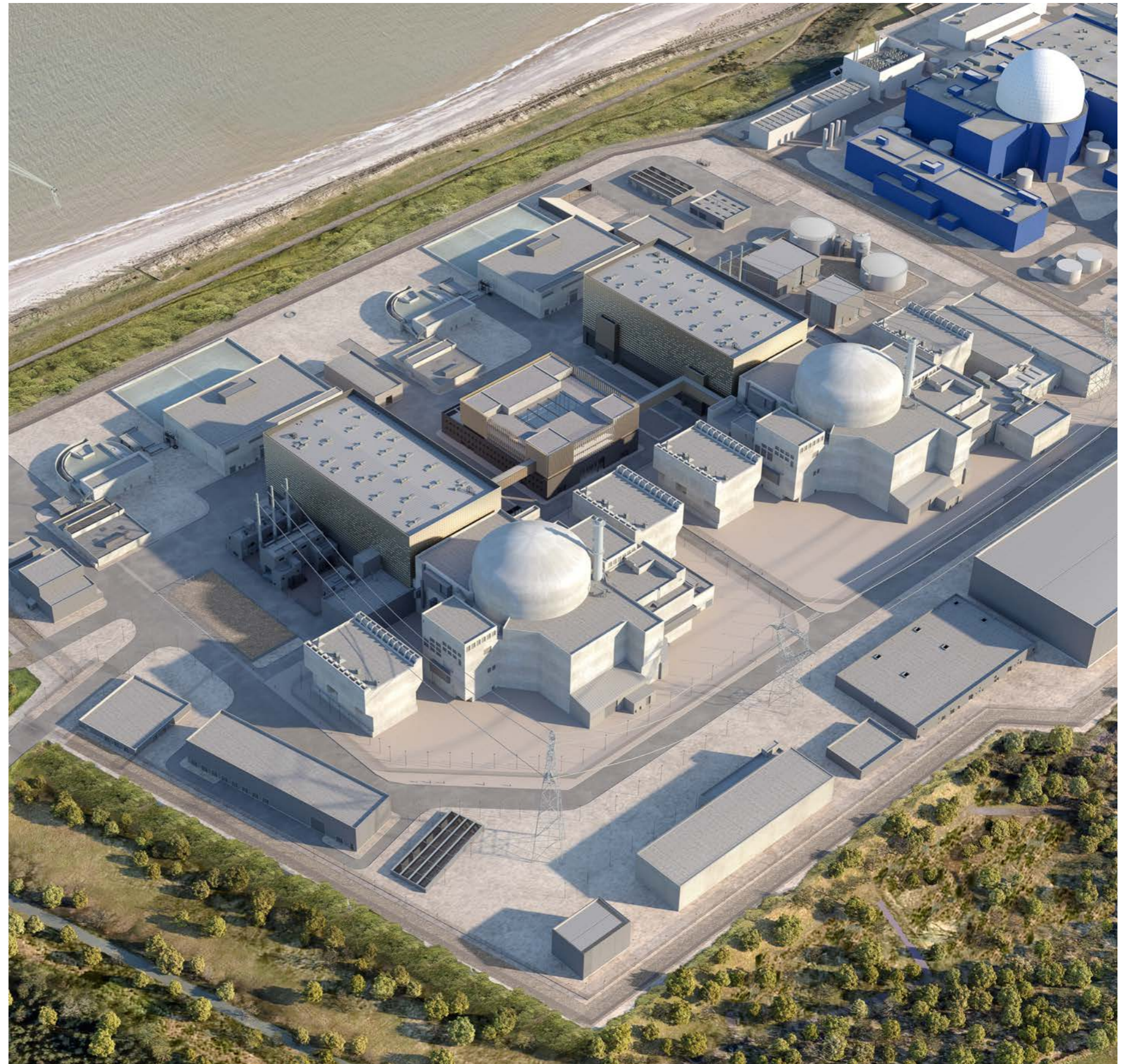
Figure 7.11: Illustrative overview of the buildings that form the nuclear island for unit 1 and unit 2 of Sizewell C
