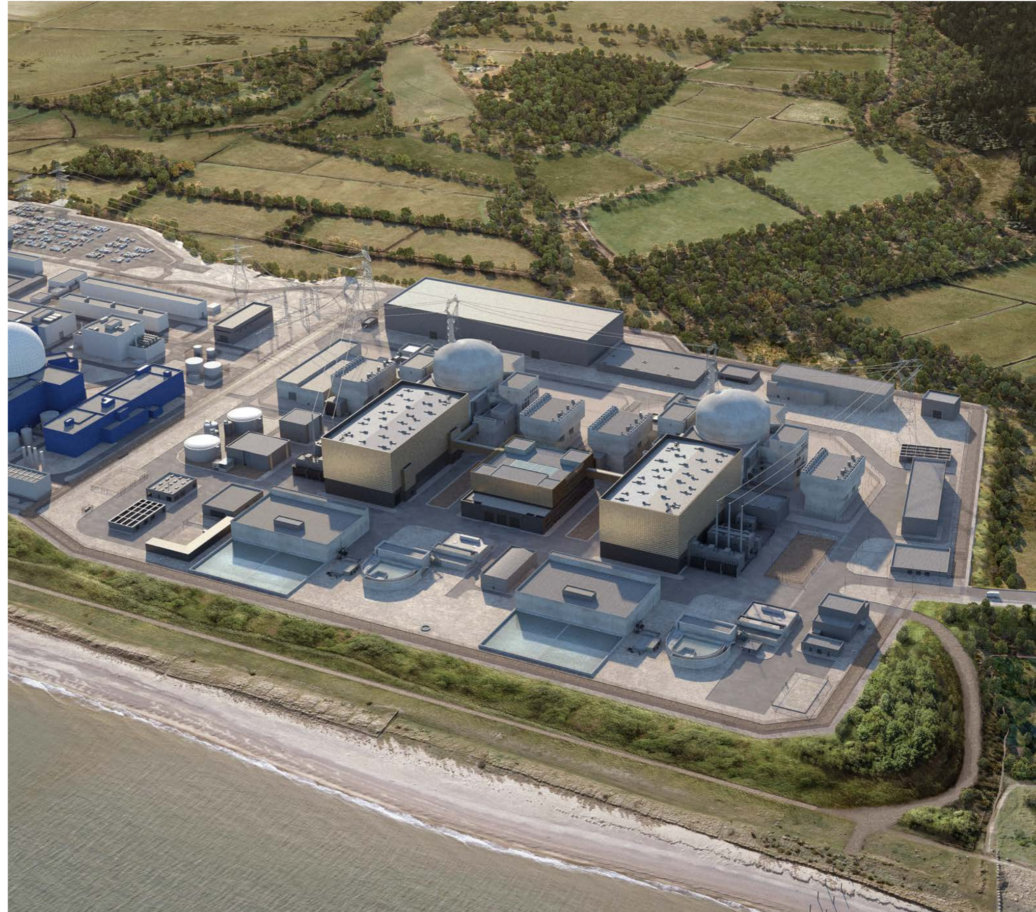
Figure 7.52: North-east aerial view of the operational service centre
