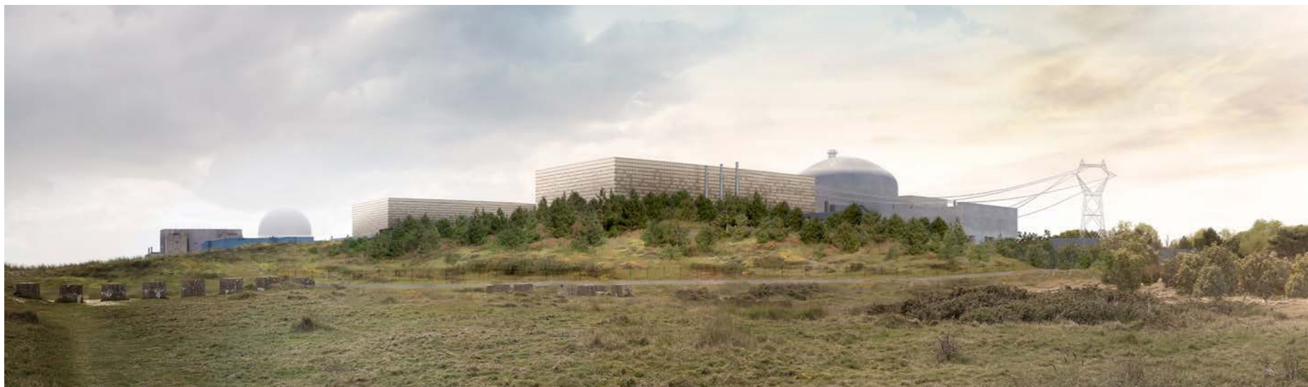
Figure 7.46: Medium bronze facade treatment to the turbine halls of Sizewell C (also right) (refer to Figure 13.10.24 of Volume 2, Chapter 13 of the ES)
