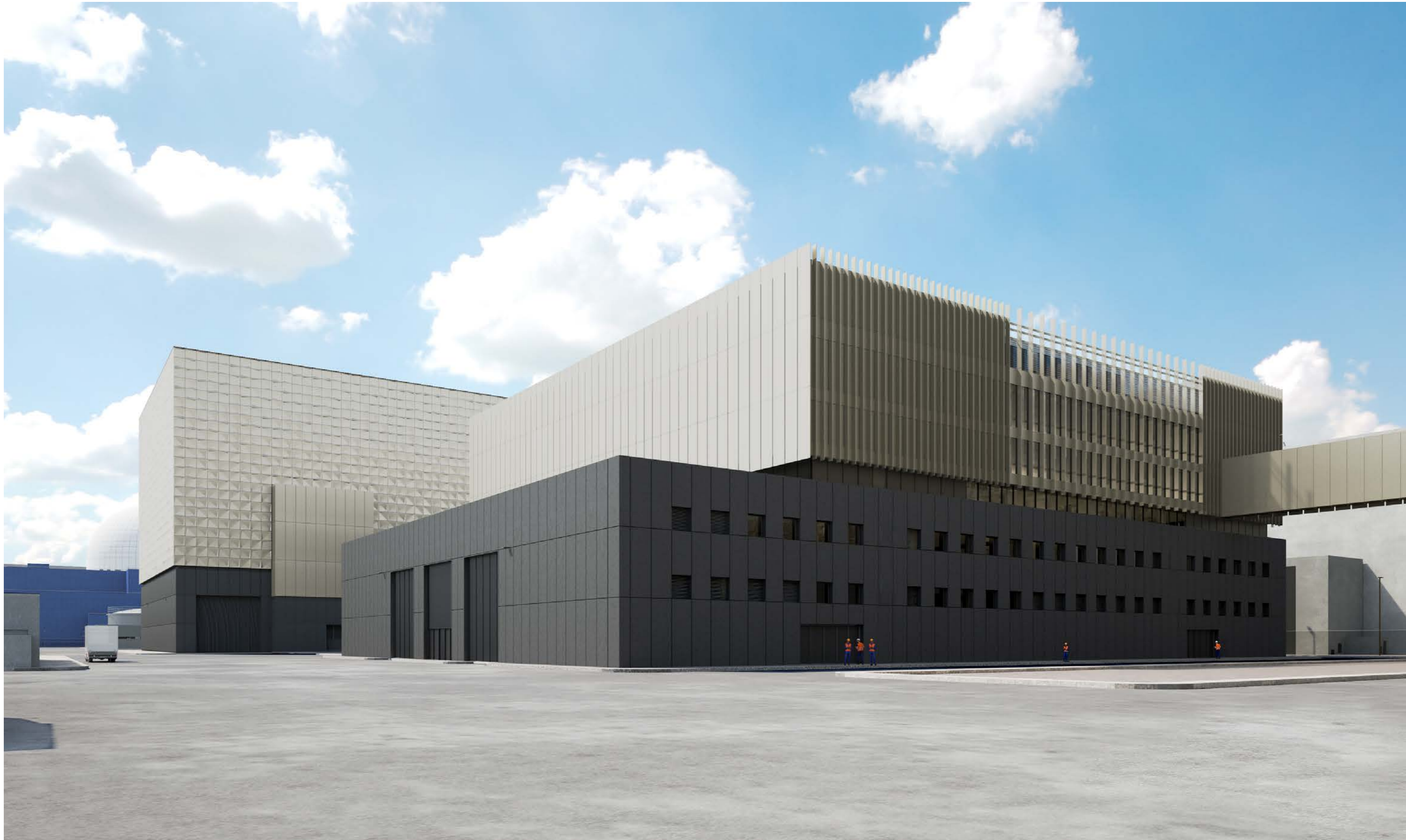
Figure 7.60: View towards the operational service centre from within the main development site
